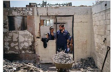
President Gabriel Boric inspecting damage site
