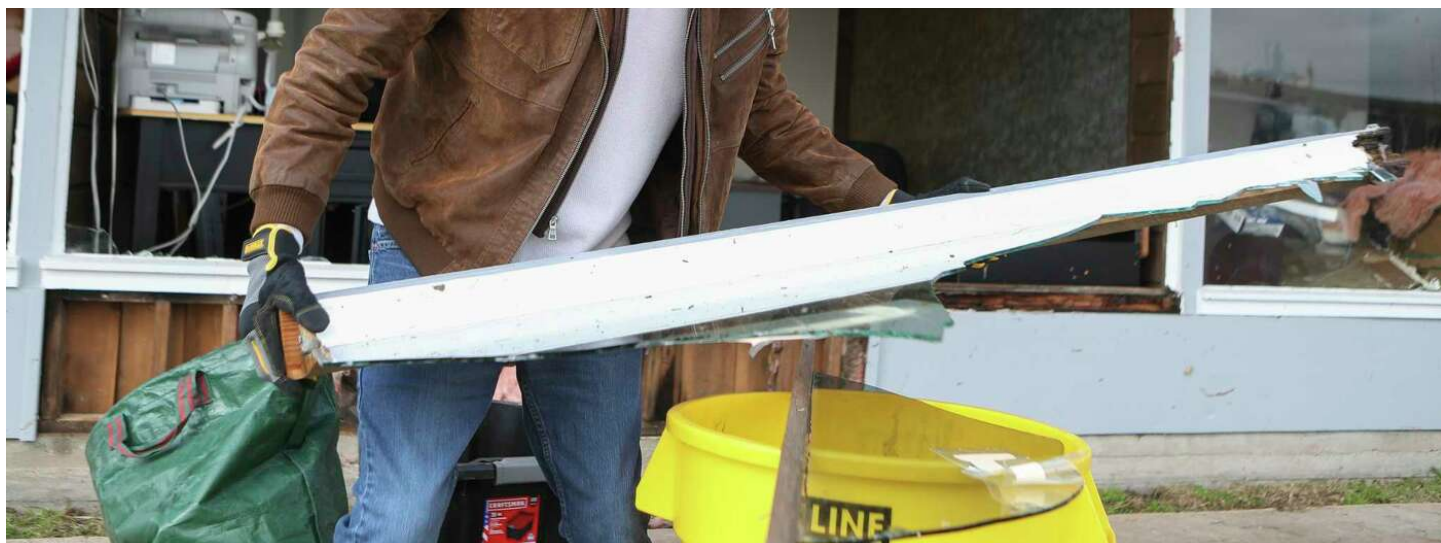
Trey Cothfan, owner of Victory Properties Inc., helps clear out debris from Tuesday's tornado, Wednesday, Jan. 25, 2023, in Deer Park.
